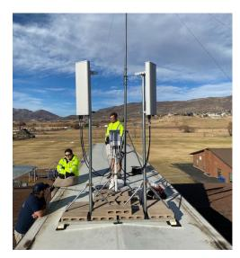
Technicians working on an installation for Wasatch School District to provide WiFi internet access using CBRS band of radio frequency.
